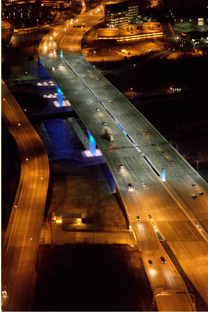
I-35 bridge in Minneapolis, MN
